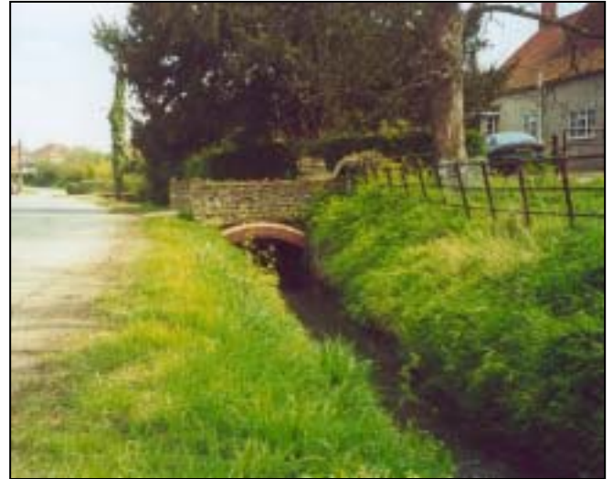
The stream on the south side of Station Street
