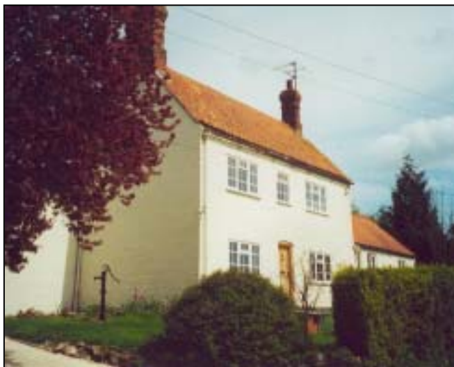
A fine example of pantiled roofing
