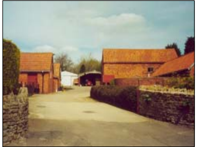
Farm buildings in Station Street
